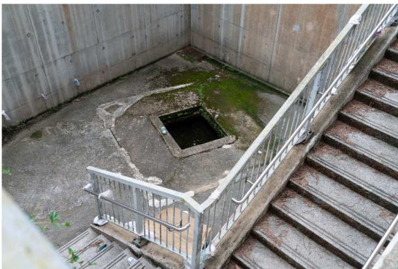
FIGURE 4. 'Well below ground', this water source now sits 2 metres below ground level after the industrial estate land reclamation project levelled the land where seashore once was.
